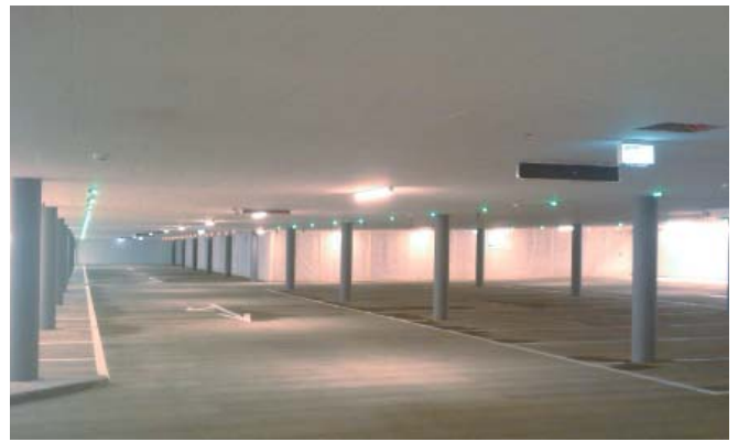
Underground car park, Wattwil (Switzerland)
